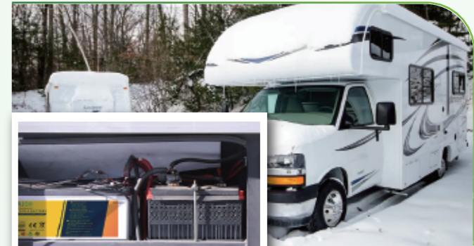
RV battery Install Model: LFP12V-200
